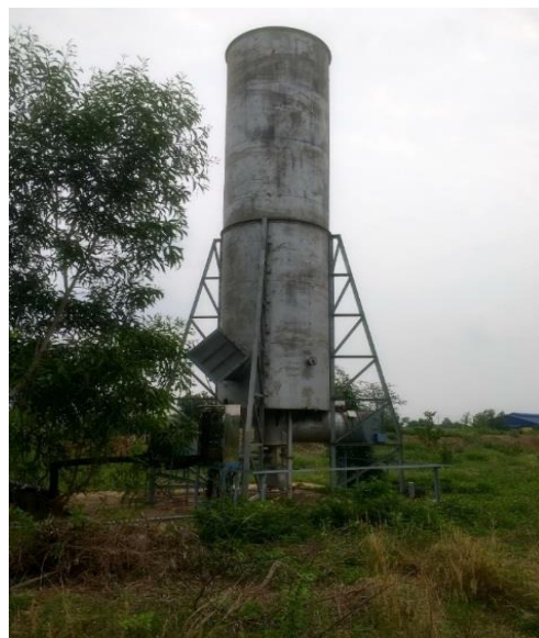
Picture 18: Gas flare at the lagoon biogas plant (tapioca factory, farm No 6)
