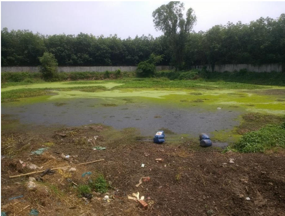
Picture 22: Lagoon in which the waste water (among others) is stored
