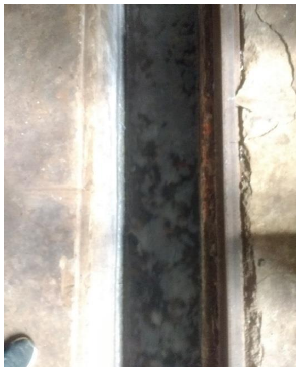
Picture 20: Channel in which the waste water is flowing from the factory into the lagoon
