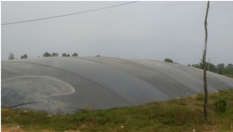
Picture 5: Electricity connection near the gas holder of the lagoon (hold up with a stick)
