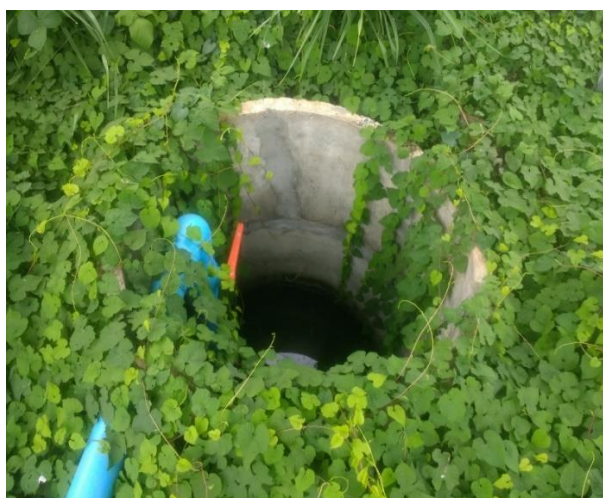
Picture 13: Condensate trap at the farm No 4
