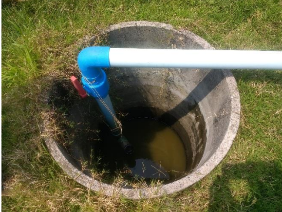
Picture 8: Condensate trap at the farm No 3
