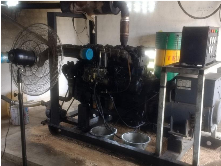
Picture 2: Genset to convert the energy in biogas into electricity
