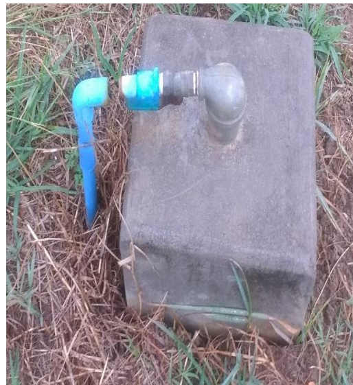
Picture 26: Tube of the domestic biogas plant (not connected)
