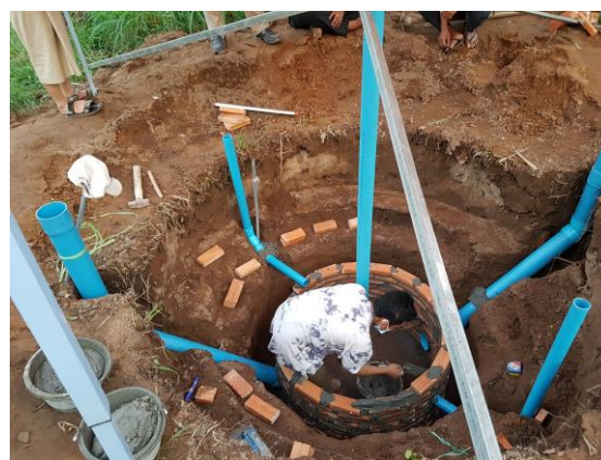
Figure 8 First masonry and piping
