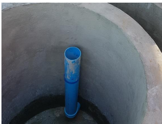
Figure 16 Outlet pipe extension
