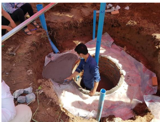
Figure 14 Pouring the foundation for water seal
