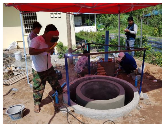
Figure 17 Work on guide poles
