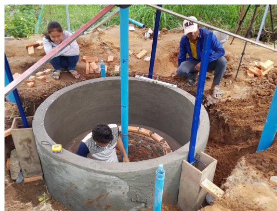
Figure 15 Constructing the inner digester wall
