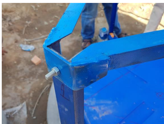
Figure 21 Angle bars connecting gas holder guides
