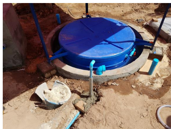
Figure 22 Gas holder in place
