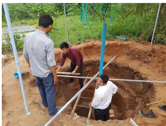
Figure 7 Excavation for a 1m 3 digester
